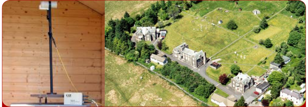
GSM-90 Overhauser Magnetometer instrumentation installed at British Geological Survey (BGS) observatory station in Eskdalemuir, South Scotland
